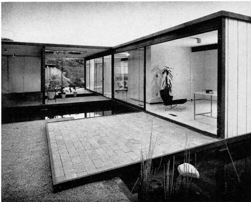
VIEW SHOWING INTER-RELATIONSHIP OF TERRACES AND POOLS. THE TERRACES ARE PAVED WITH THE NEW DAVIDSON PAVING BRICK.
