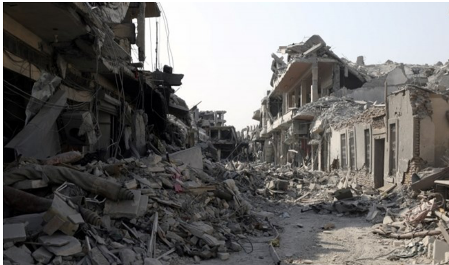
A view of a damaged site is seen in Raqqa, Syria September 16, 2017. REUTERS/ Rodi Said
